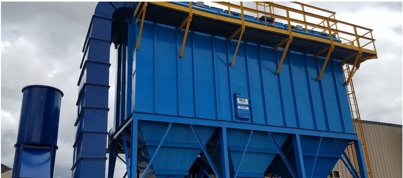
Industrial dust collection system used to capture particulate emissions from the production process.
