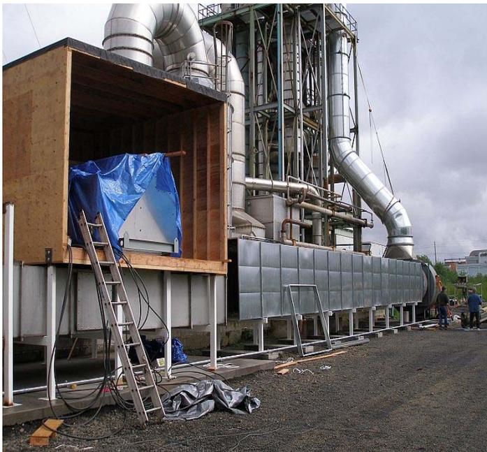
Fig. 6: Injection, DBD based Cold Plasma system. Power rating: 36kW. Main air flow is 150,000 m<sup>3</sup>/hr, injection air is 25,000 m<sup>3</sup>/hr
