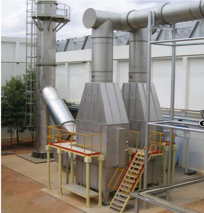
Fig. 5: Flow through, PCR based Cold Plasma system
